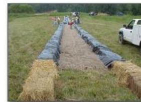
Figure 15. Lower portion of the treatment ditch
