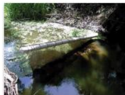
Figure 29. Particle curtain in a canal
