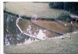
Figure 30. Particle curtains clarifying the input to a pond
