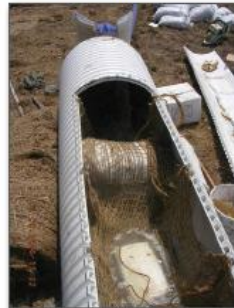
Figure 20. Split pipe with polymer blocks
