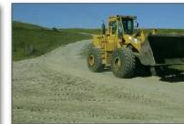
Figure 13. Road dust after applying polymer flocculant
