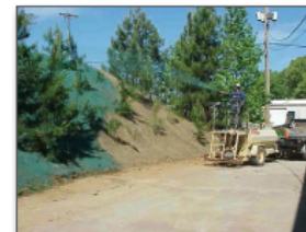
Figure 5. Hydroseeding the slope
