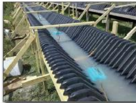
Figure 17. HDPE treatment ditch liner
