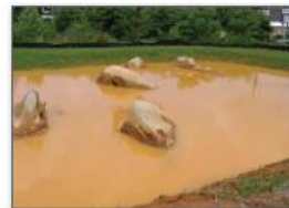
Figure 40. Sediment pond before BMPs were installed
