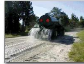
Figure 11. Water truck applying dissolved polymer flocculant
