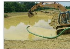
Figure 14. Sediment basin to be dewatered
