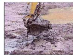
Figure 36. Removing stiffened sediment from a sediment basin
