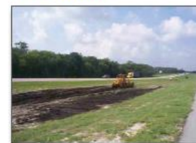
Figure 37. Recycling sediment along a highway
