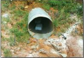
Figure 39. Polymer block in a construction site culvert
