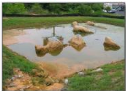
Figure 41. Same pond after BMPs were installed
