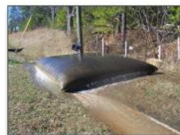
Figure 34. Sediment bag and its treatment ditch
