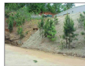
Figure 4. Slope covered with floc collection matting
