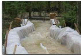
Figure 8. Large mixing ditch
