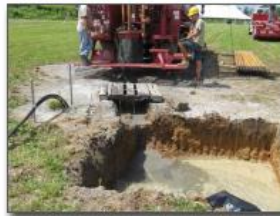
Figure 7. Drilling rig and settling pit
