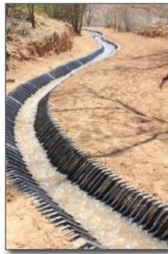
Figure 18. In-ground treatment ditch
