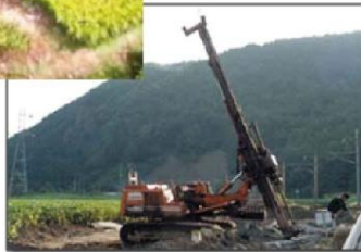
Bulbous Micro-pile Method
