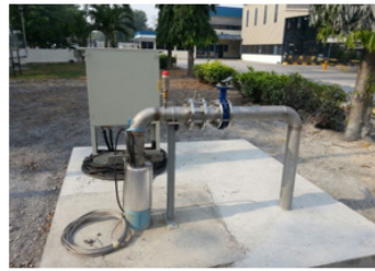
Completed groundwater station (this well produces about 0.5 mld)
