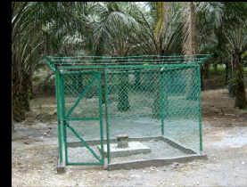
A completed well
