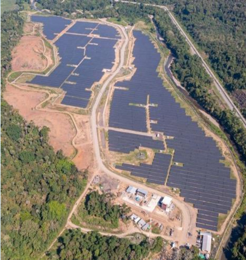
Solar PV Power Plant with the 26.8 Megawatt, currently the largest in Indonesia.
